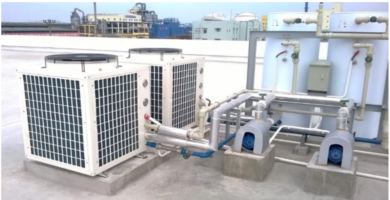
Installation of Hot Water Supply Units for Building
