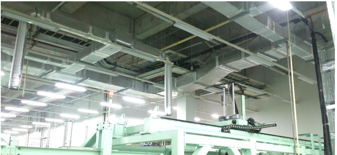
Installation of Ventilation system
