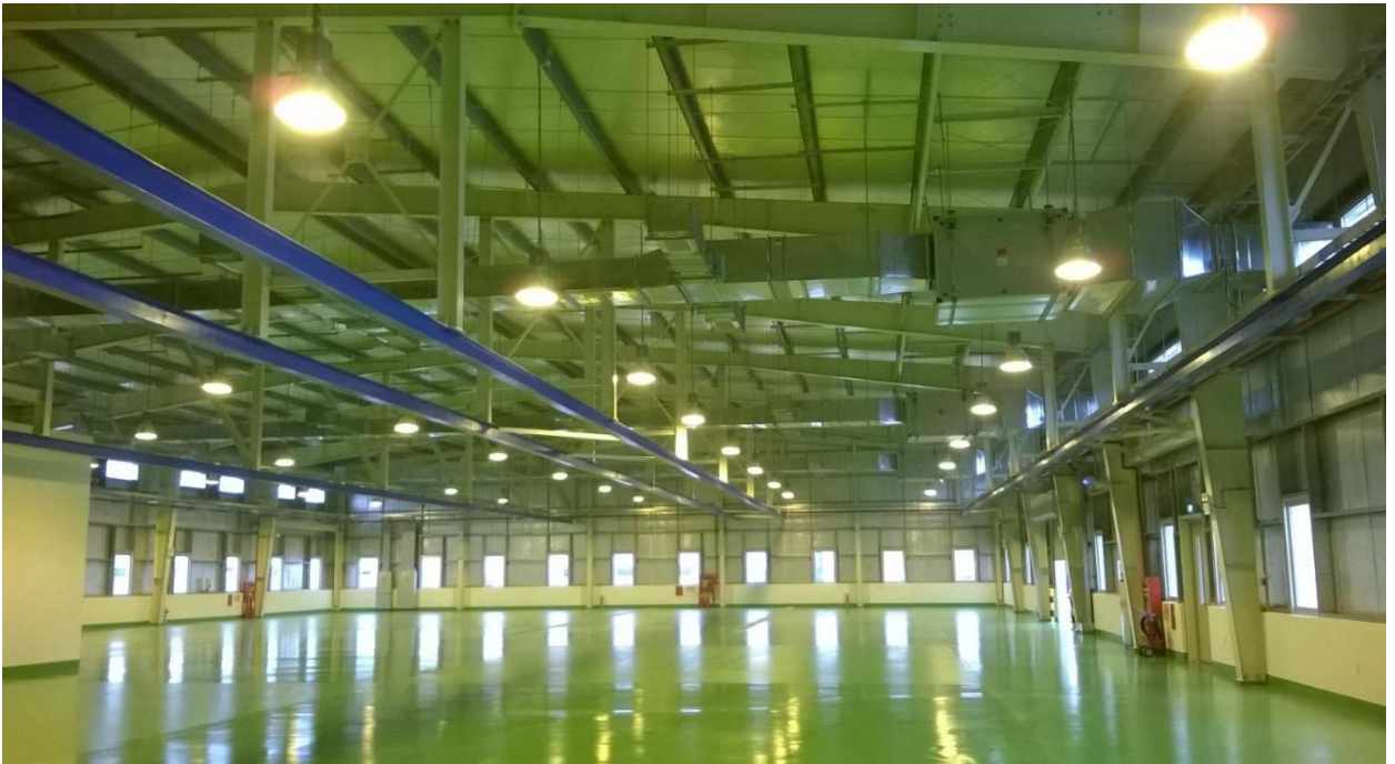
Installation of Electrical in Factory
