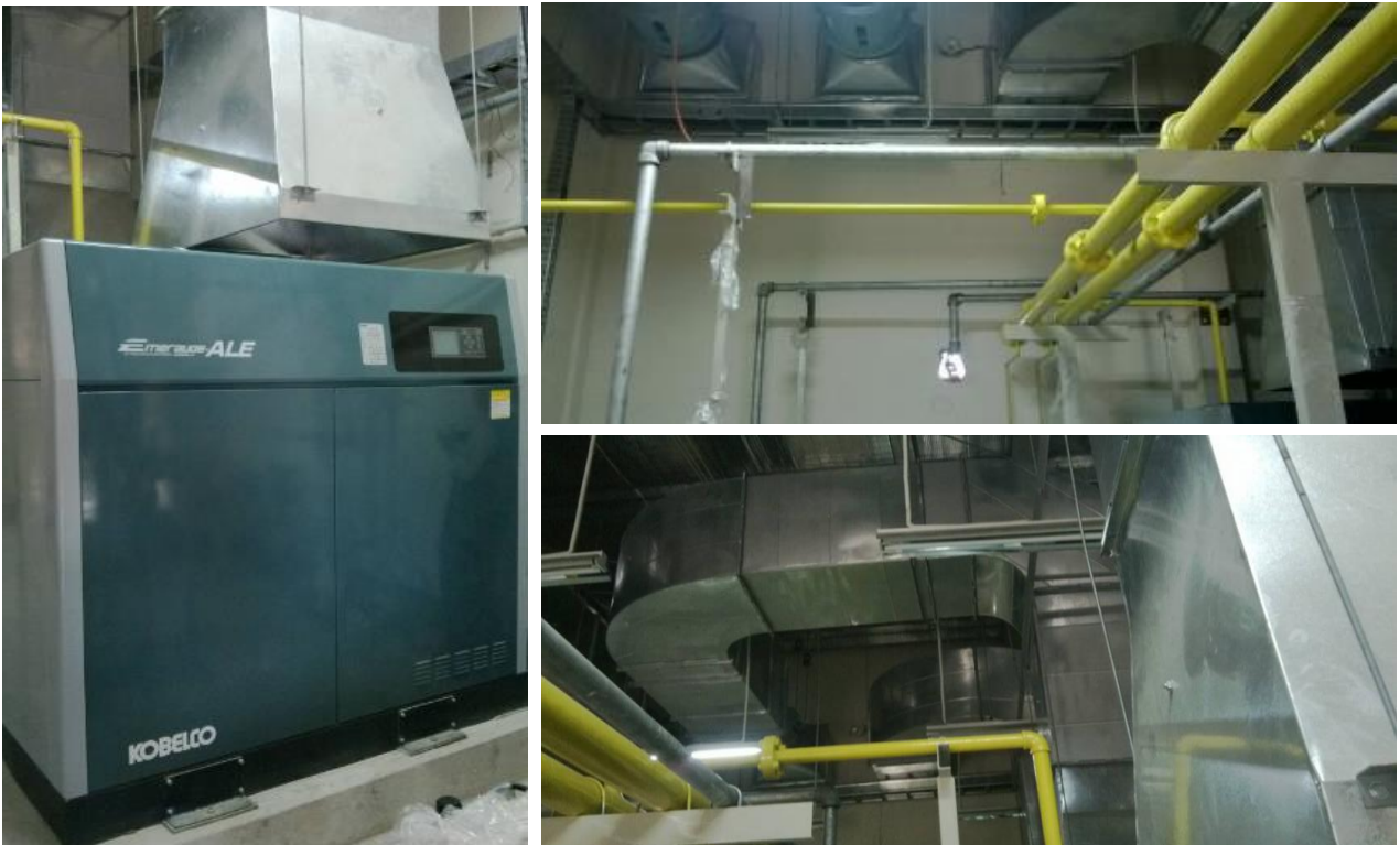
Installation of Compressed Air System
