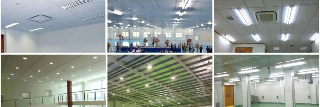
Installation of Electrical System in Office Building
