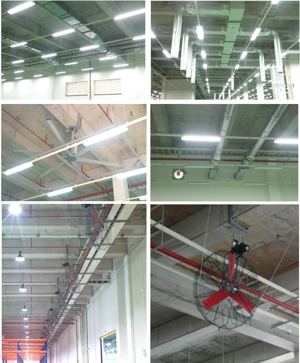
Installation of Ventilation system
